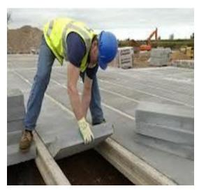
To seal the floor, the whole floor area should be grouted with a nominal **4:1** sharp sand/cement mix as soon as possible after the fixing of floor beam and blocks are completed. This should be done by brushing the grout over the floor with a stiff broom (after the surface has been well 'wetted') so that the grout penetrates the joints (block to block & block to beam) to provide a rigid construction.
